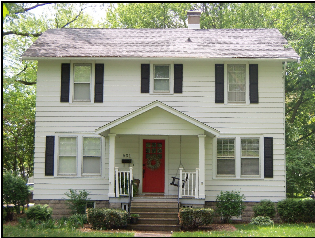
2014 – Metal storm door removed; original wood door remains
